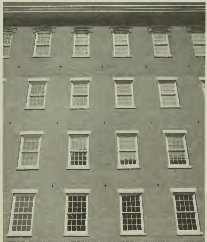
Figure 9. The window solution represents an important advance in the way in which aluminum windows can be designed to capture more fully the appearance of historic windows in larger buildings. Right photo shows wood sash in bottom row and aluminum in the upper three rows. Photos: Jim Higgins ©
